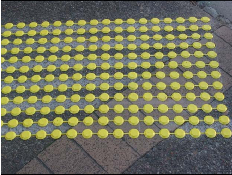
TACTILE HAZARD WARNING INDICATORS
