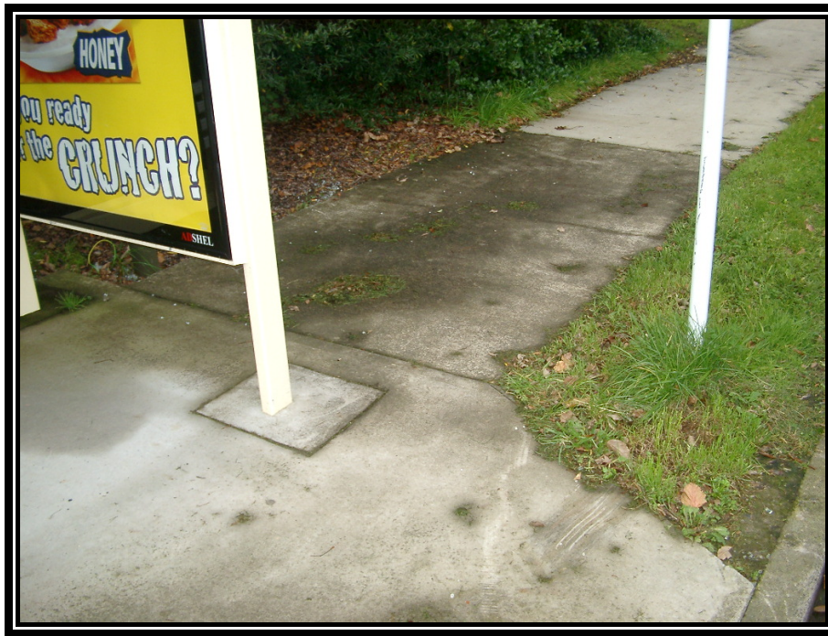
Photo 6 - An example of a poorly located bus shelter and pole hinders pedestrians, wheelchair users and pushchair users alike.
