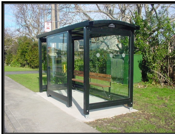
Photo 10 - Good shelters have high visibility for passengers, no hiding spaces for undesirables and promote passive surveillance.
